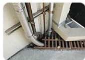
Bendable vacuum-insulated pipe is more forgiving of existing ductwork and other components.
