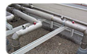
Rigid vacuum-insulated pipe often is used for the outside portion of distribution systems.
